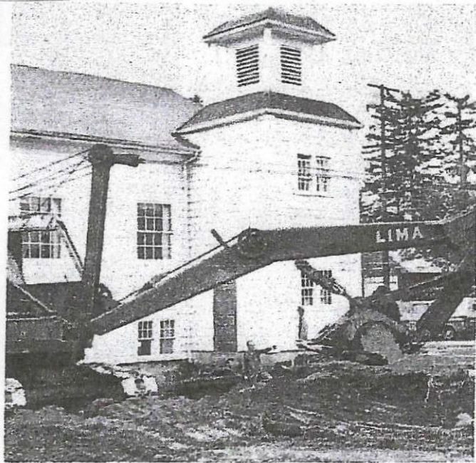
Excavation of the basement
